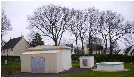
Station de pompage
